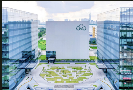
CMC TELECOM CMC Data Center HCM - HN
